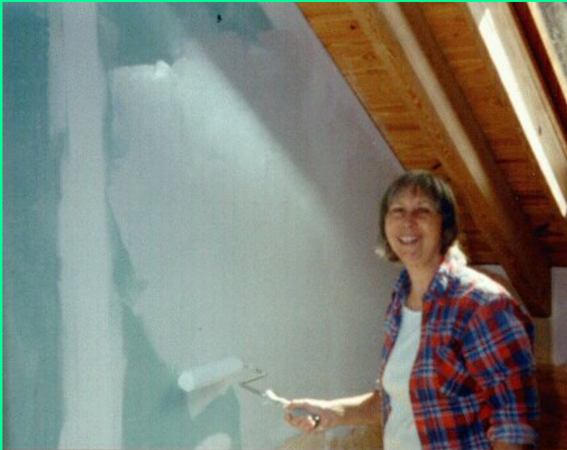
2nd floor bathroom Rosemary is painting the 2nd floor green-board.
